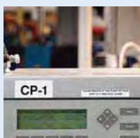
Control Panel and Electrical Panel Labels
